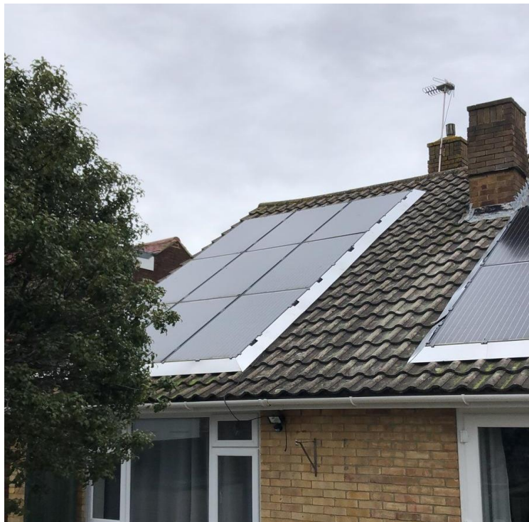
A SolaSkirt Silver installation on a black framed solar PV system.
